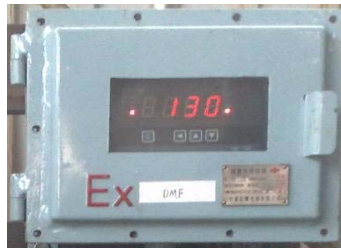
▲XMT-100 防爆型数显仪 (是给 XMT-100 数显仪加装防爆盒，可装于现场)
